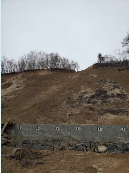
Slope restored – location previously was large gully
