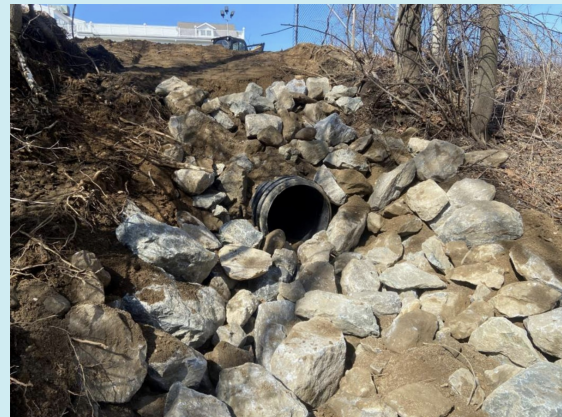
Permanent outflow pipe for eastern tennis courts
